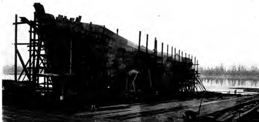
Ship No. 1 on the ways and ways prepared for a second vessel alongside at the Standifer-Clarkson yard, North Portland.
